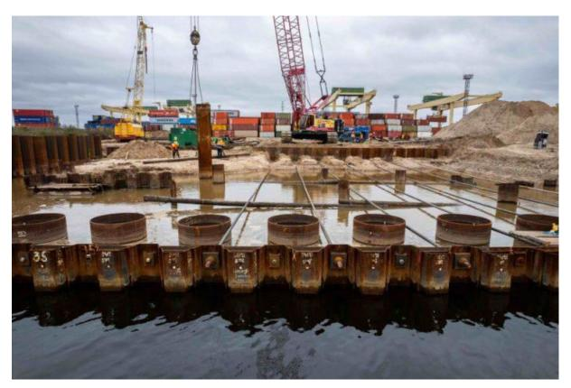
Construction works are underway in Kundzinsala at the Baltic Container Terminal (BCT), the largest box terminal of the Port of Riga, with the underwater works for the construction of a new berth section having been completed.
