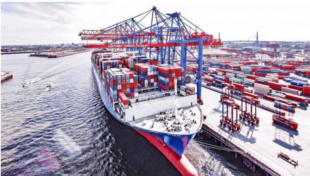
Container Terminal Tollerort (CTT)
