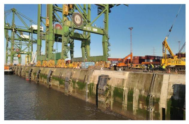
The Port of Antwerp-Bruges has recently enhanced the bollard capacity at PSA Antwerp's Noordzee Terminal by upgrading four bollards from 150 tonnes to seven new 250-tonne bollards.
