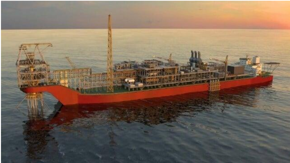
Woodside's Sangomar FPSO (Illustration courtesy Woodside)
