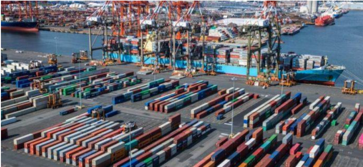
Maher Container Terminal
